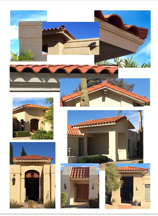
Exterior Walls and Columns: All homes have stucco walls. The finish texture is mainly lace in a medium to heavy pattern. Some homes have modernized with a sanded stucco finish. Few homes have full-height stone veneer wrapped columns/pilasters or stone veneer on portions of front façade and garage doorjambs.
