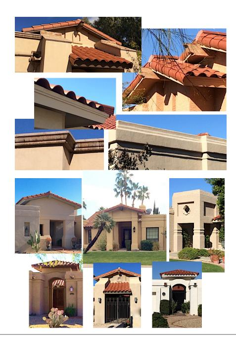
Exterior Walls and Columns: All homes have stucco walls. The finish texture is largely lace in a medium to heavy pattern. Some homes have applied a fine, sanded stucco texture. Few homes have full-height stone veneer wrapped columns/ pilasters or bays on portions of front façade and garage door surrounds.
